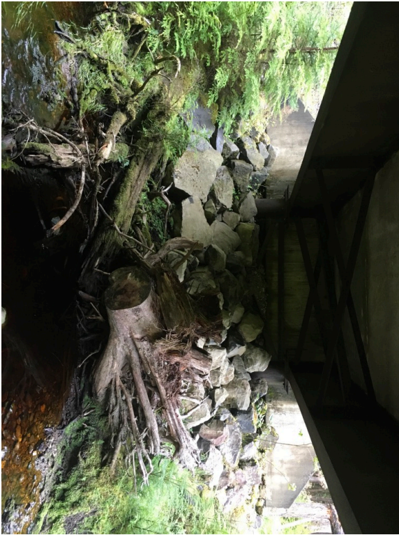
Left Bank Abutment when facing downstream
